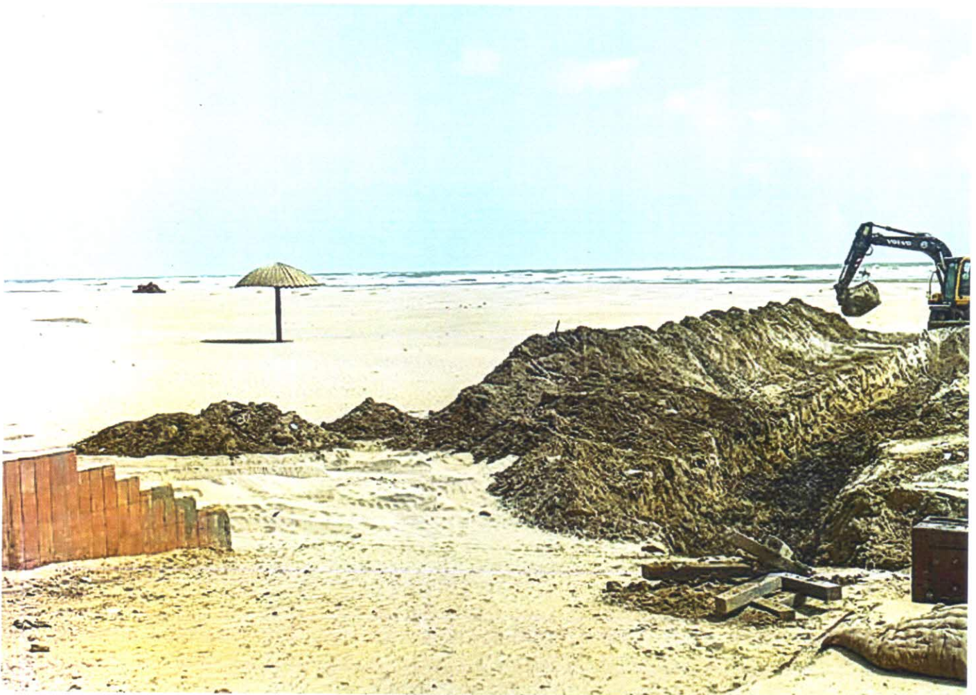
Construction work in progress at Clifton beach.—Fahim Siddiqi/White Star
